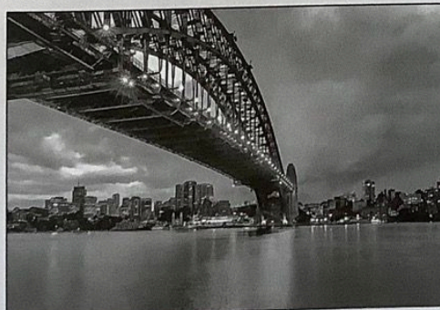
Sydney Harbour Bridge
